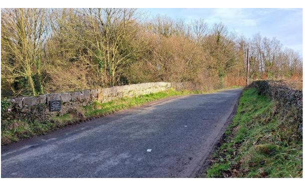
Plate 10.8 . Kilnahown Bridge (*NIAH 14933012 and RPS 52-05 Offaly & 825 Laois*) looking S. The low parapet walls have ashlar block coping stones. The bridge spans the River Barrow which is the boundary between Counties Offlay and Laois
