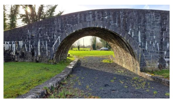
Plate 10.14 . Looking W beneath Blackhall Bridge from the infilled canal. The former towpath can be seen as a kerbed area on the left
