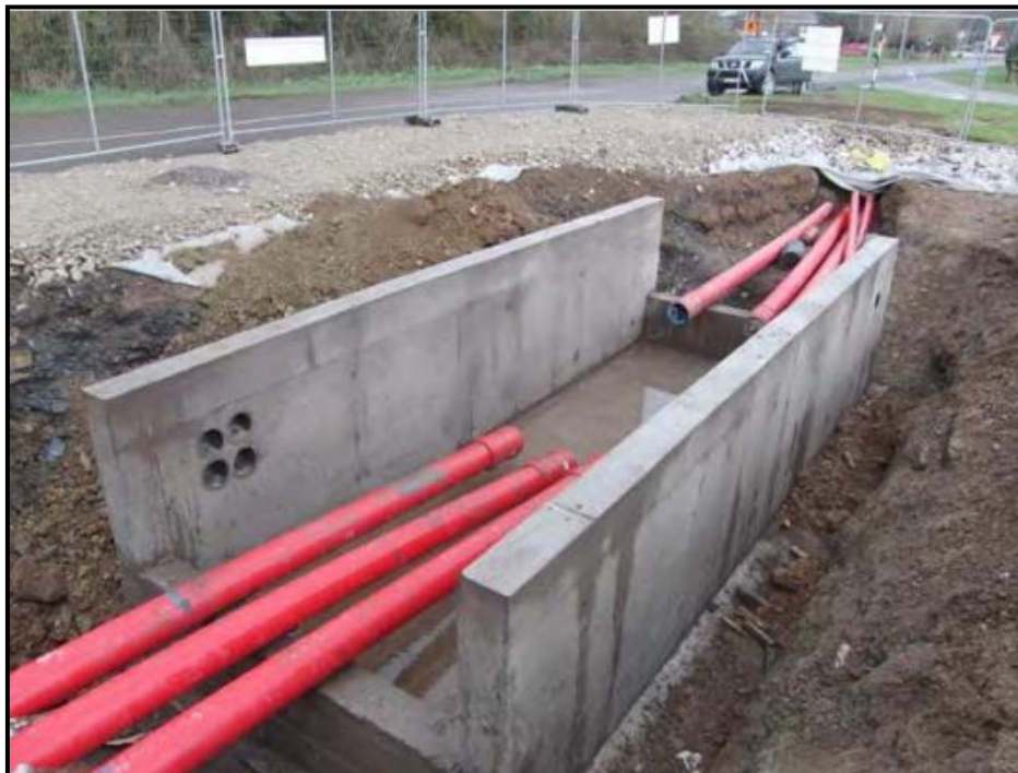
Figure 3-4 Joint Bay Installation
