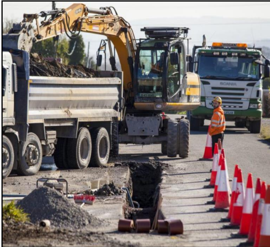
Figure 3-1 Photograph of Trenching in Public Road
