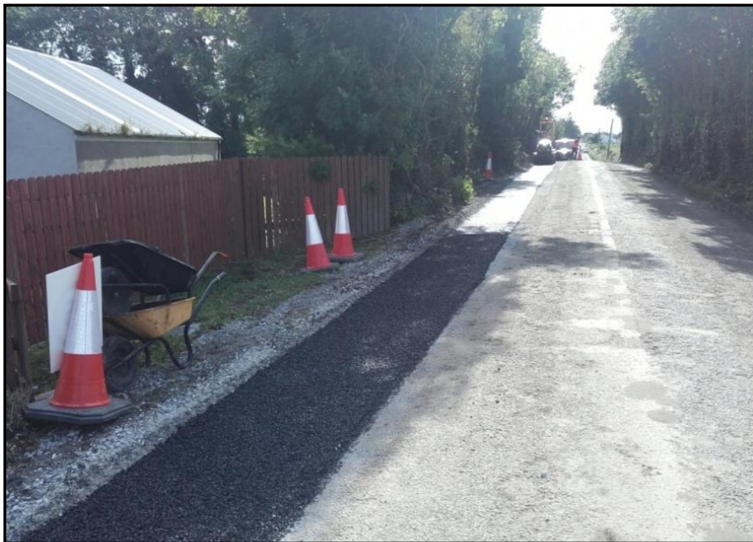
Figure 3-3 Temporary Road Reinstatement
