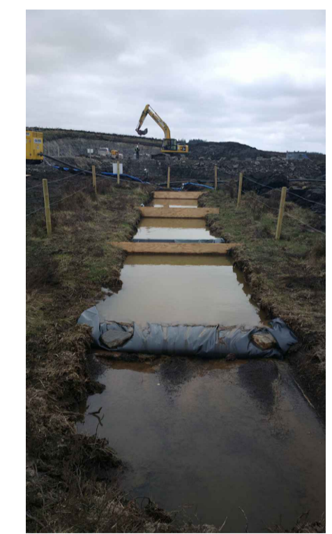
COMPLETED SETTLING POND SYSTEM
