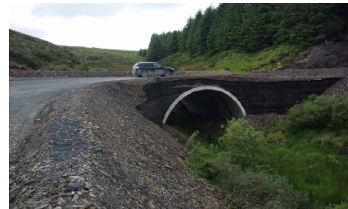
BOTTOMLESS ARCH CULVERT CROSSING
