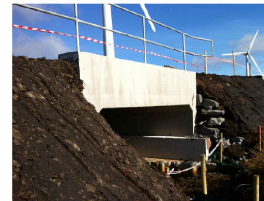
BOTTOMLESS BOX CULVERT CROSSING
